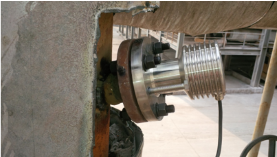
FIGURE 2. AL-CAR-K TYPICAL INSTALLATION
